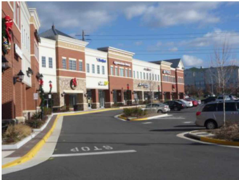
Figure 20: Parapet walls with cornice treatments are used to disguise flat roofs
