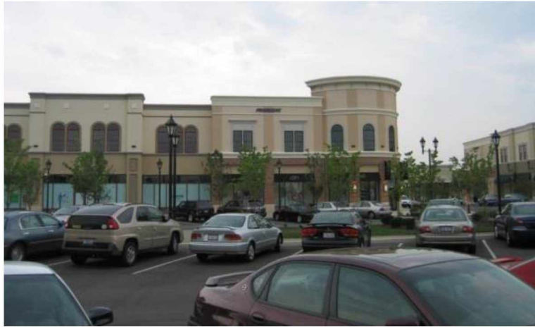
Figure 19: Roofline changes shall be aligned with corresponding wall offsets and/or material or color changes
